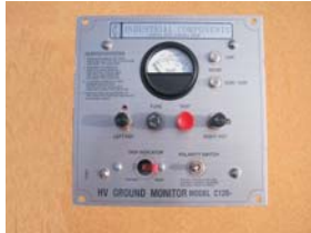
High Voltage Ground Monitor
